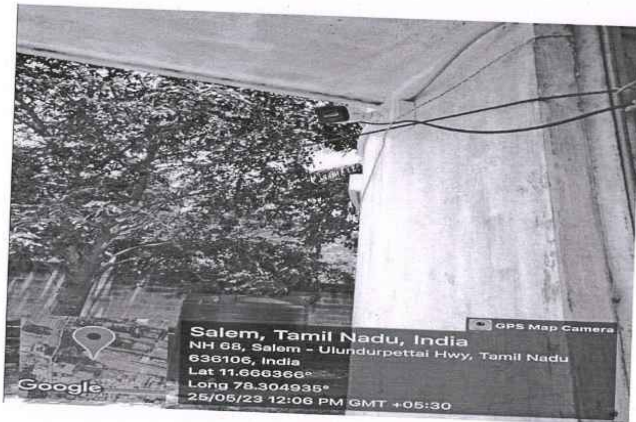
HOSTEL FRONT CAMERA
